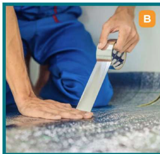
Tape all floor insulation joints.
