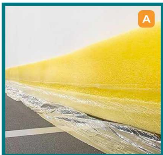
Edge perimeter foam insulation.
